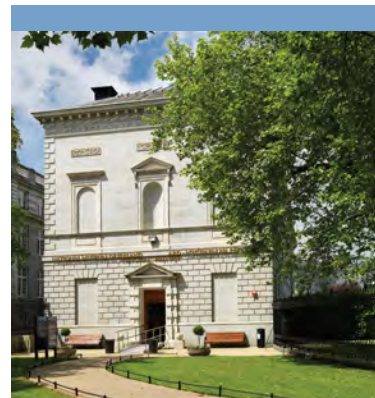
Natural History Museum, now fully accessible at ground floor level.
