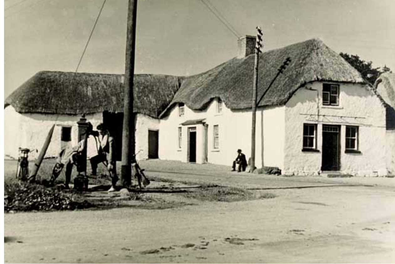
The coming of electricity to the countryside was ongoing from the late 1920s. Thatched houses at Lusk, Co. Dublin, photographed in 1943
